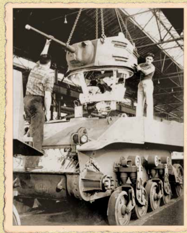
In the production line at the Massey-Harris plant in Rancine, a turret is hauled on a Stuart tank.
